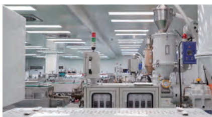
C Plant : Dedicated To Conical Tubes
